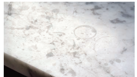
A quality marble polishing compound can be effectively used to erase light etching on POLISHED marble and other calcite-based stone surfaces.
